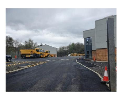
The site is now almost 1,000 square metres larger and includes a new office facility; new hardstanding; drainage; a state-of-the-art four bay fleet workshop; new material storage and an external fuelling area. This fuelling area is separate but linked to the depot providing options for easier, safer refuelling and provision for new EV chargers to meet the needs of our modernising fleet.
